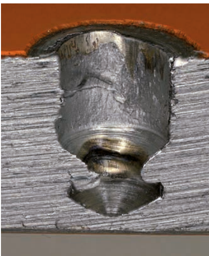
Steel base material after 10 years of exposure to sea water and pull-out of the X-BT fastener. The hole appears clean and no evidence of corrosion is visible.
